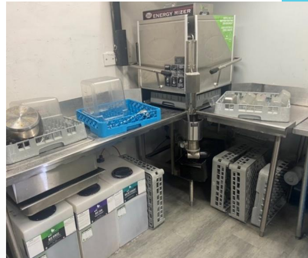
Installation of commercial dishwasher
